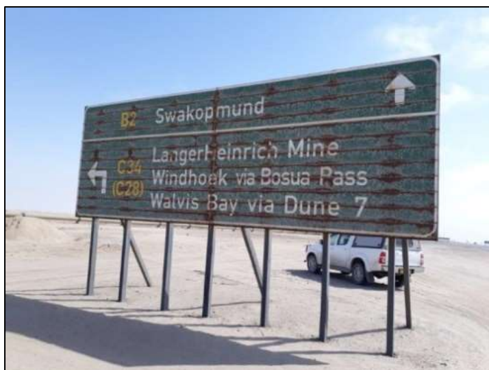
Figure 7: Corroded Sign on B2 Road
